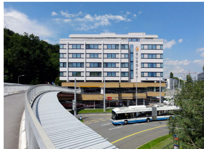
Umbau Boardinghouse, Zürich
